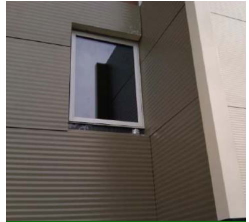
Fiberglass window in renovated façade Photo courtesy of WinnCompanies
